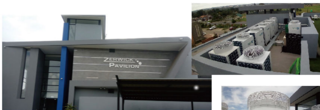
Name: Zerwick Pavilion Location: Kempton Park ,GT Series: Heat Pump Scale: 185 kw
